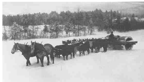
Breaking the roads with the snow roller, winter of 1925.
